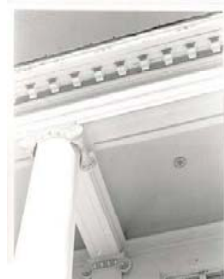
DENTIL WORK ON THE ROOF SOFFIT AND THE TOP OF A COLUMN.
